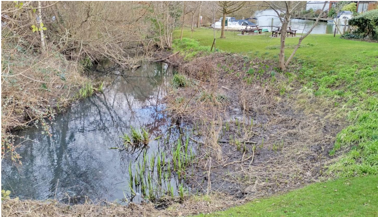
Christchurch Ditch outlet location showing silt and vegetation accumulation, downstream of the closed section of the culvert at Heron Island.
