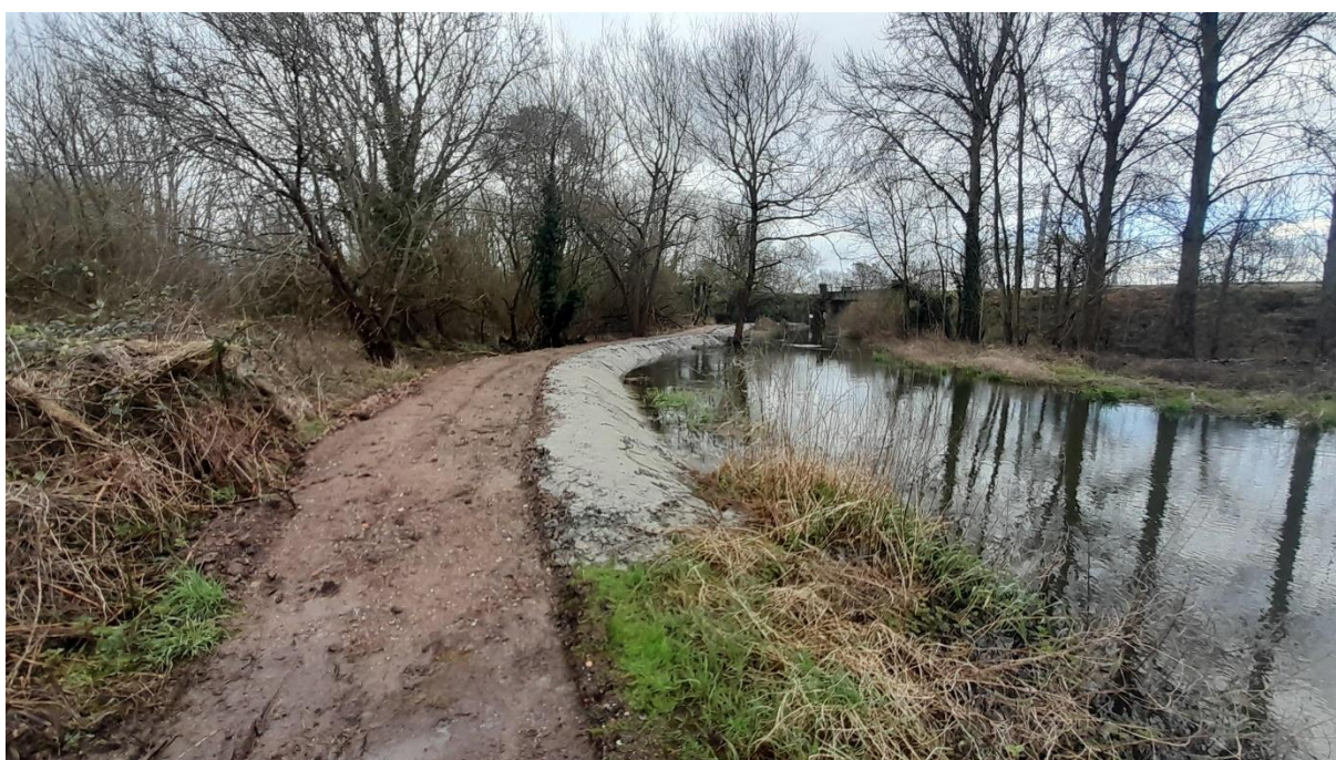
Temporary repairs to damaged banks, Holy Brook, west of Briscoe's Bridge
