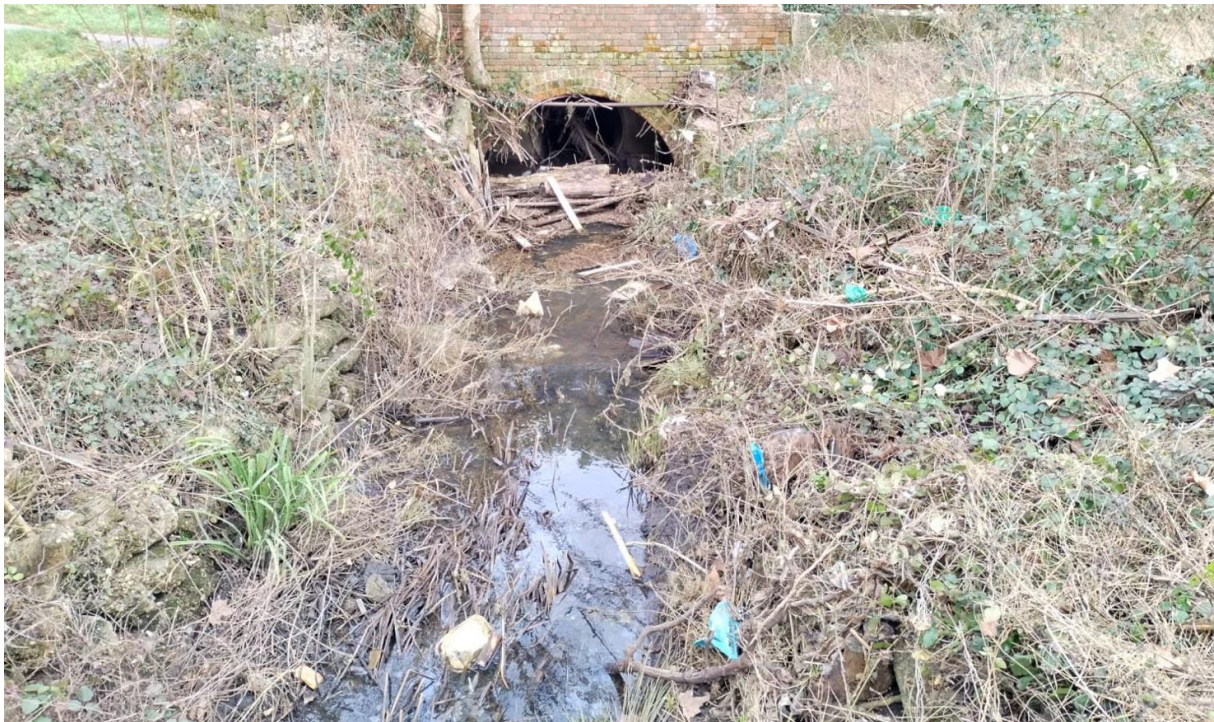
The accumulation of excessive woody debris along the channel leading to the culvert entry upstream of Heron Island.
