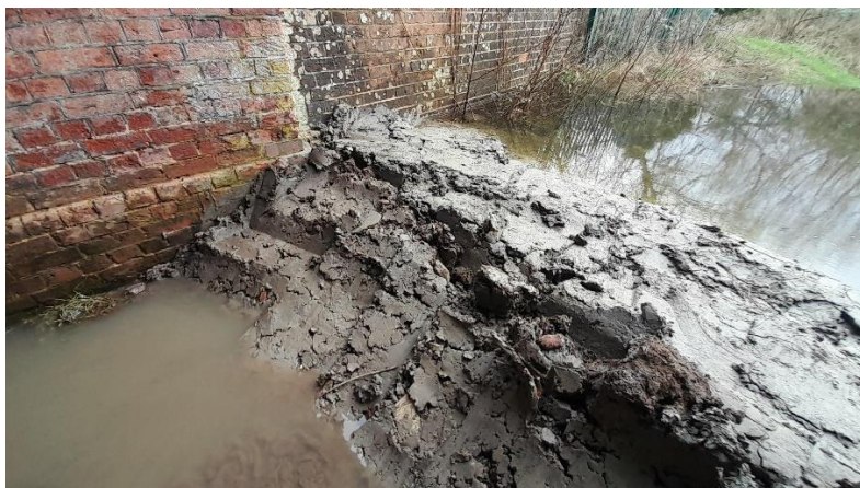
Temporary clay bund under Briscoe's Bridge, Southcote
