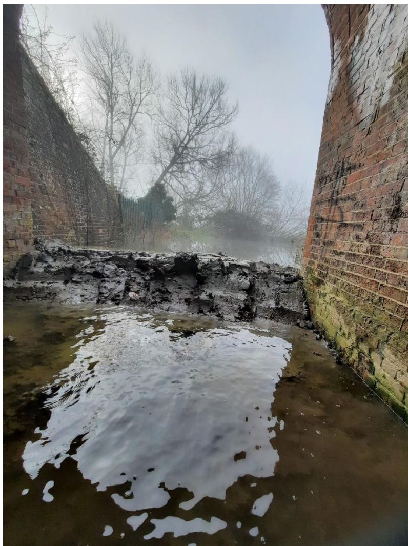
Photo provided by local resident, 8 th March 2024, showing effectiveness of temporary bund holding back water from floodplain under Briscoe's Bridge
