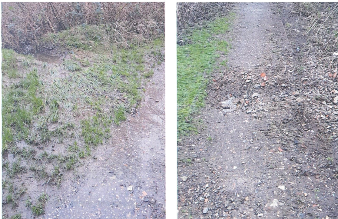
Damage to post-2014 bank and path repairs near Holybrook overbridge, Southcote
