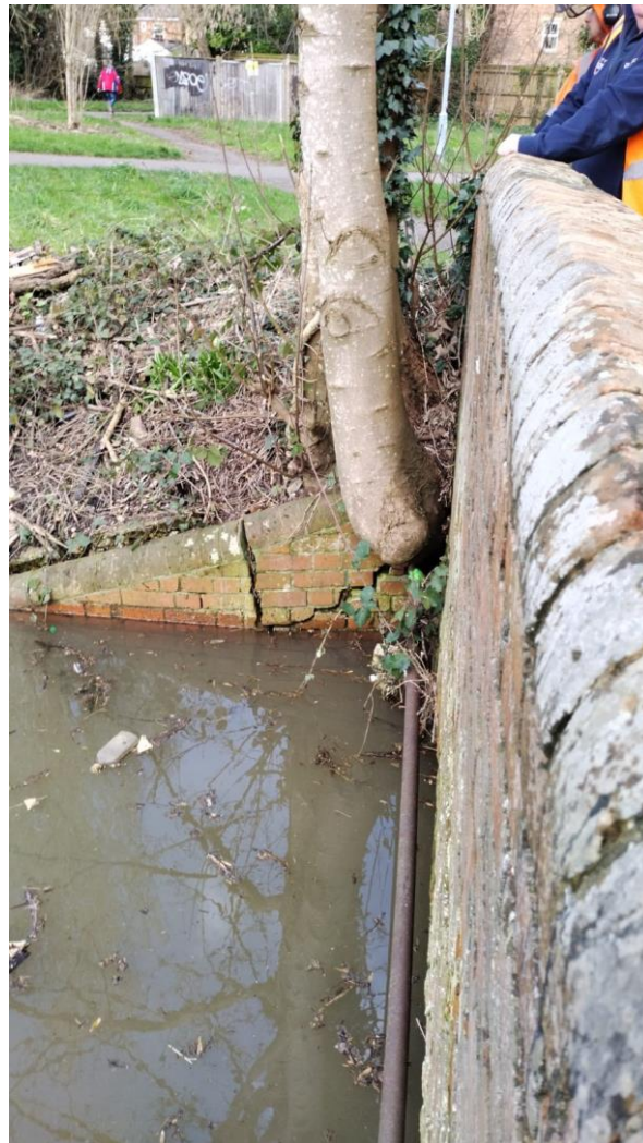
Partial blockage of culvert by woody debris and tree growing into footbridge, eastern end of Hills Meadow, Lower Caversham
