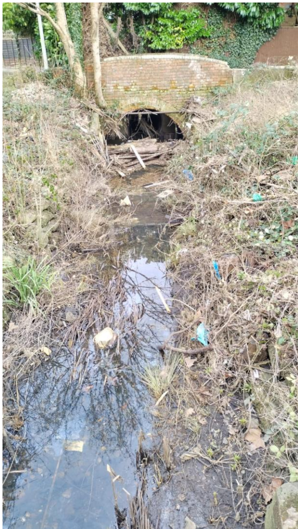
Partial blockage of culvert by woody debris and tree growing into footbridge, eastern end of Hills Meadow, Lower Caversham
